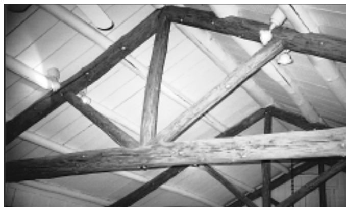
Original cabin beams
