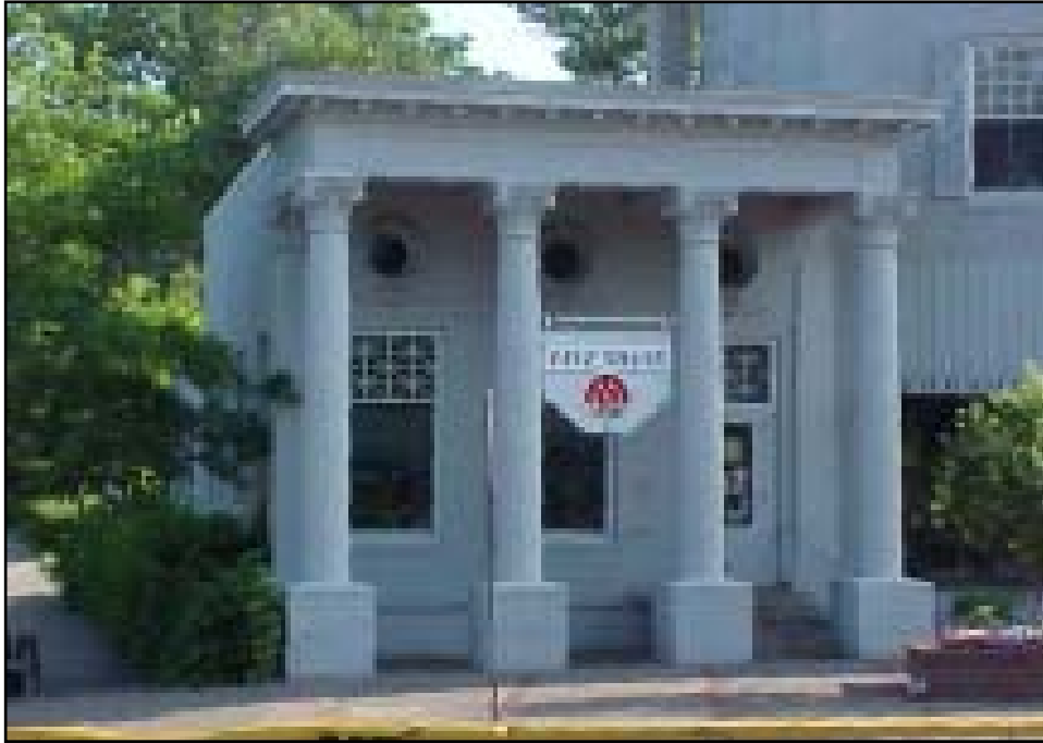
20. Wayzata State Bank Building, 305 Lake St. E.
