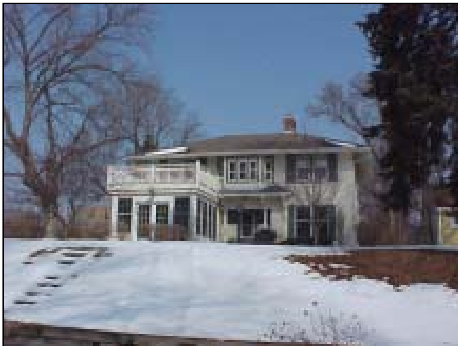
13. Ramaley House, 121 Grove Ln. E.
