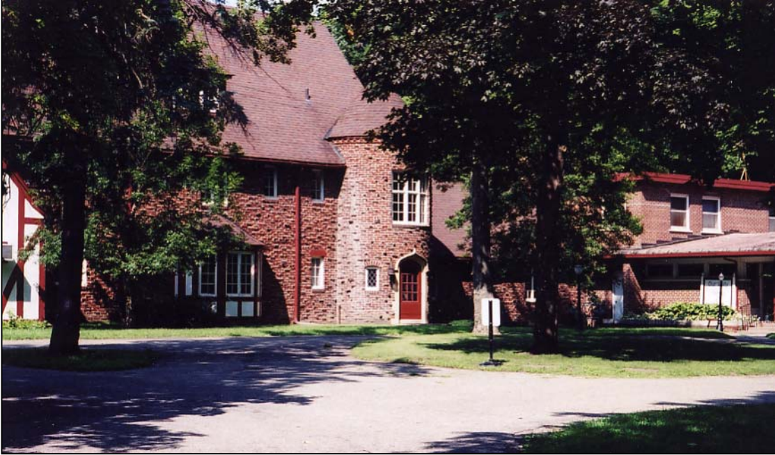
26. Arnao House, 1201 Wayzata Blvd.
