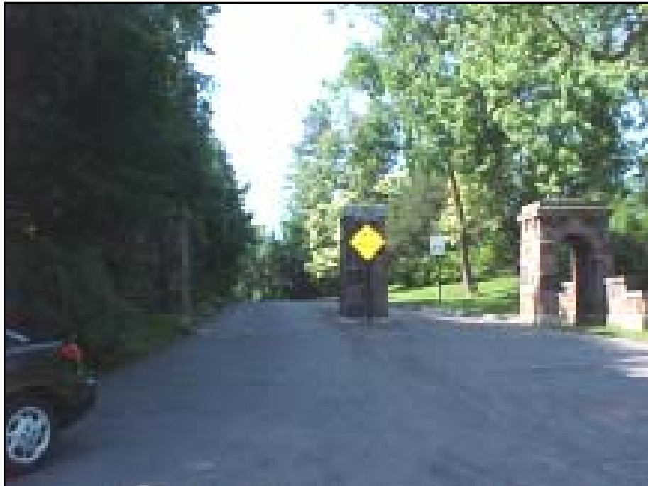
29. Harrington Farms Gate, Harrington Rd. at Ferndale Rd.
